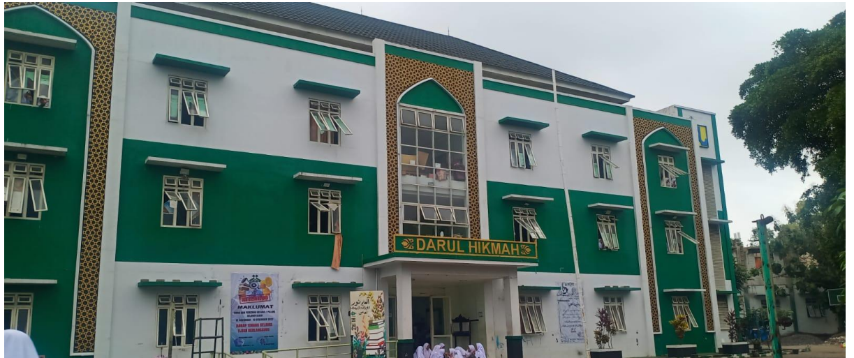
Boarding School Building
